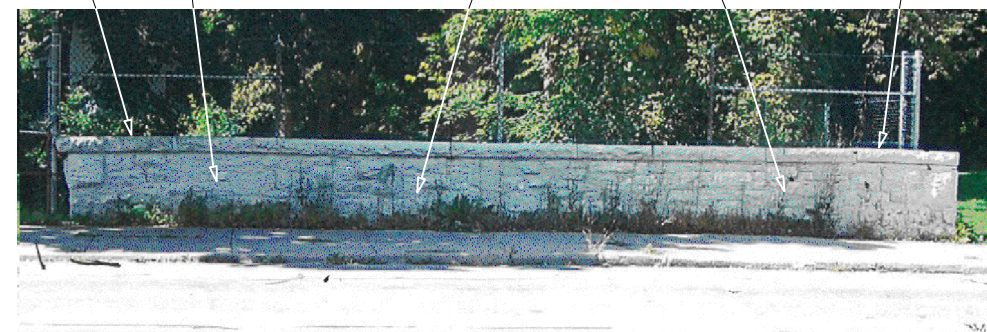
SOUTH END WEST PARAPET/BARRIER WALL NORTH END
