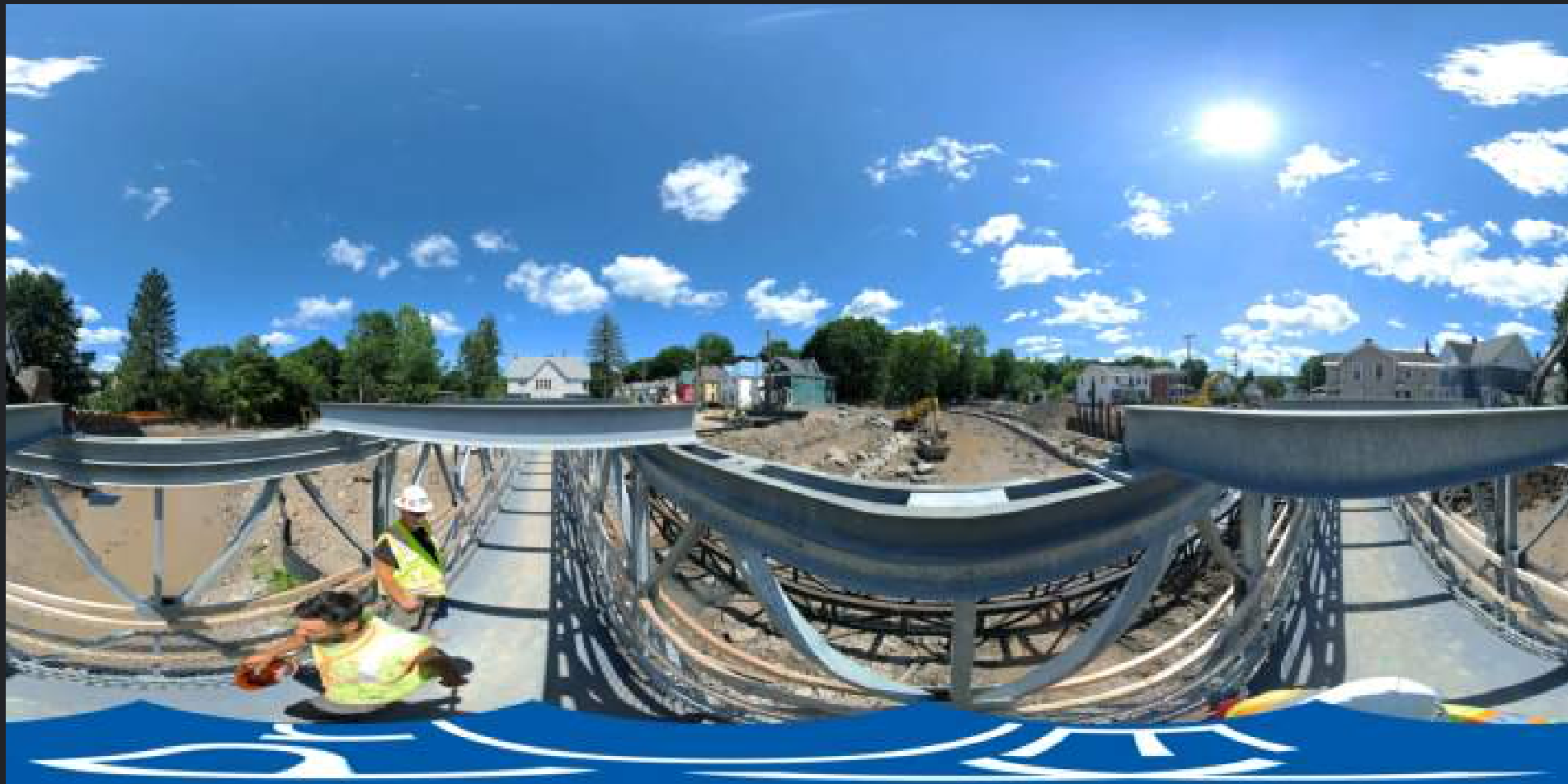
Location E – During Construction
