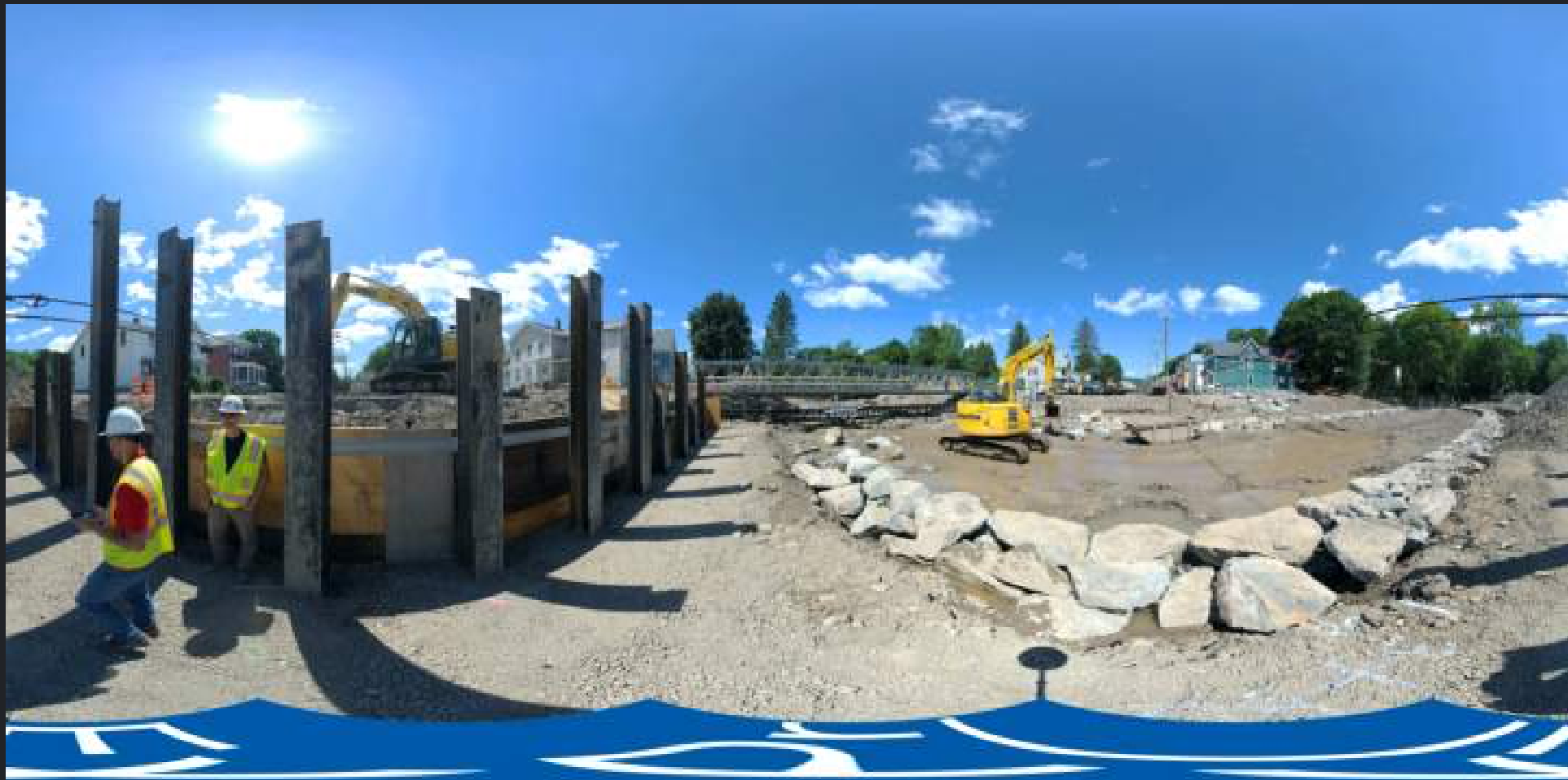
Location A – During Construction
