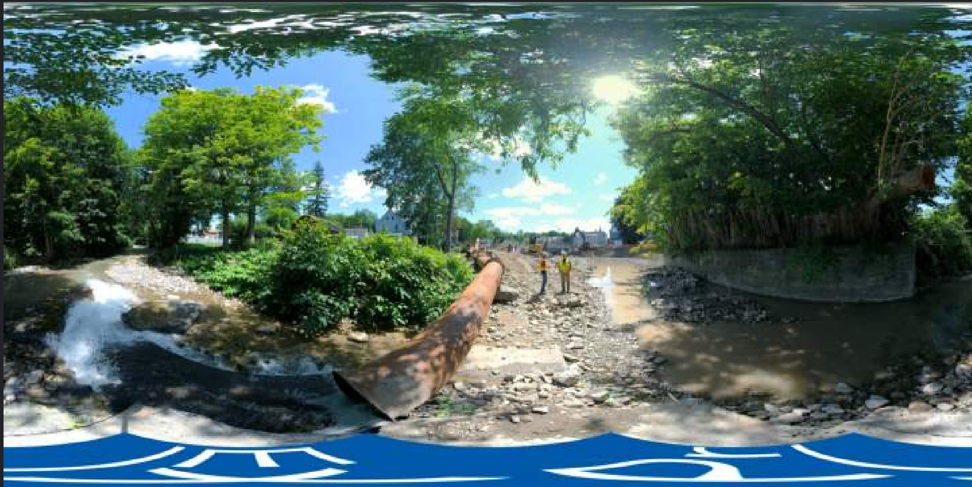
Location H- During Construction
