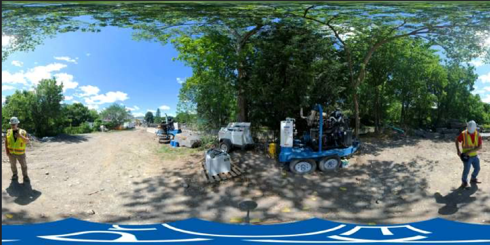
Location G1 – During Construction
