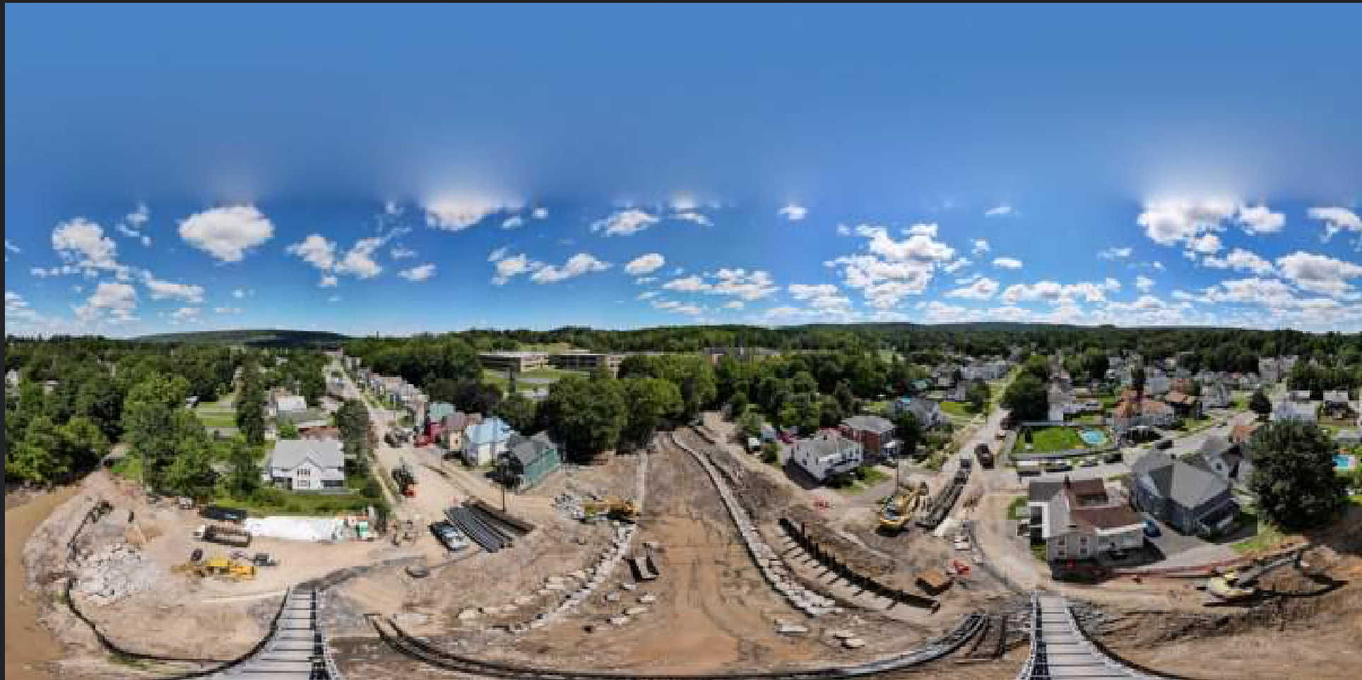
Drone View Looking Upstream – During Construction
