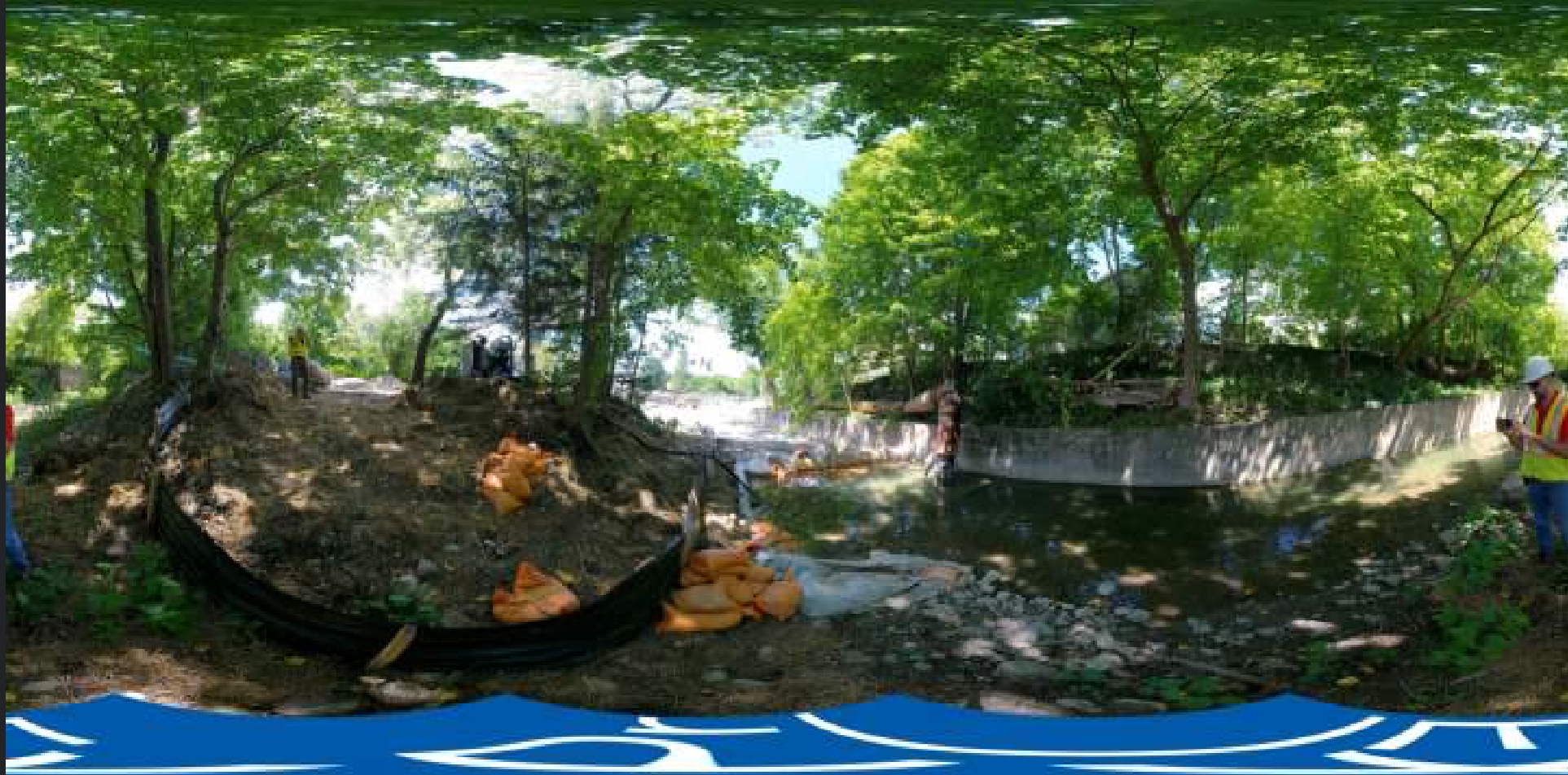
Location G2 – During Construction
