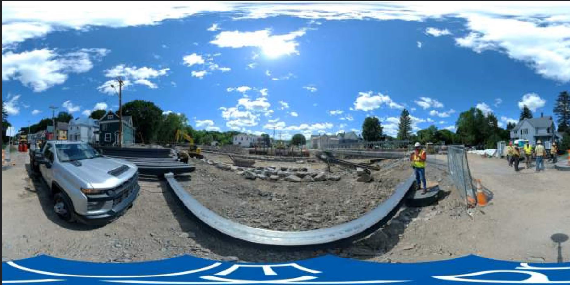
Location F – During Construction
